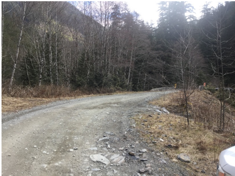
Approach from Right Bank when facing downstream
