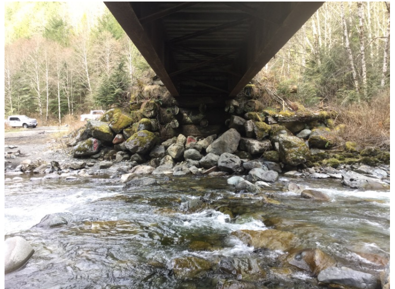
Right Bank Abutment when facing downstream
