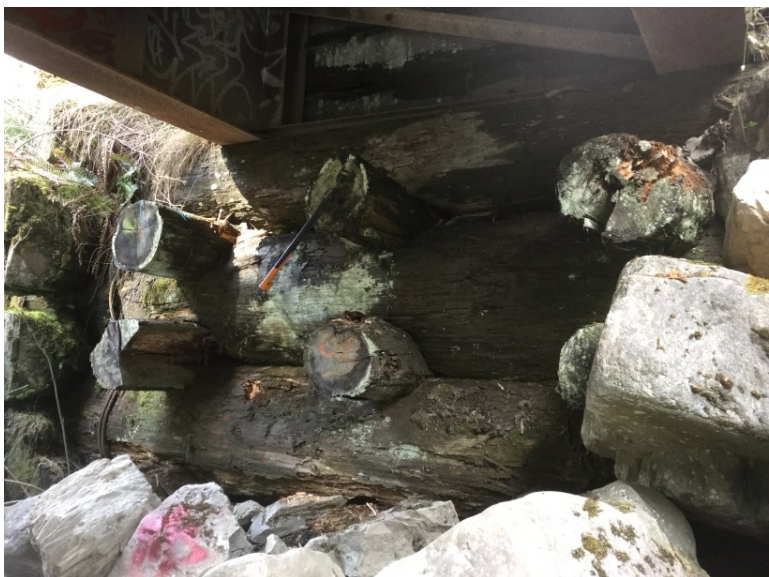
Crib condition at right bank
